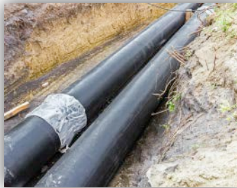
Pipeline Leak Detection System
